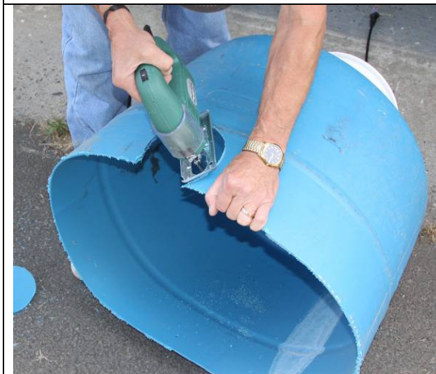
Figure 19. Cutting the 5.75 in. hole with jigsaw.
