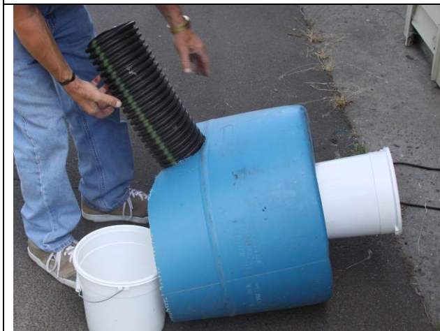
Figure 21. Insert the 6 x 16 in. drain line collar section 2-3 rings into barrel; affix firmly with adhesive, inside and outside of barrel. This needs to be solid.
