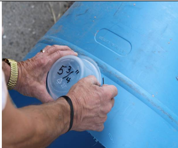
Figure 18. Scribe a 5.75 in. hole onto bottom edge of barrel for the 6 in. drain line collar section. Note: a smaller hole is cut for the 4 in. drain line design.
