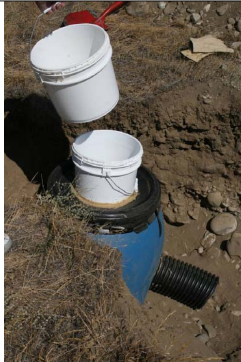
Figure 26. Finished burrow chamber, top buckets, and collar. Unit is being installed.
