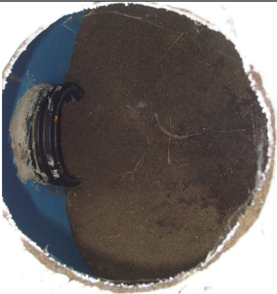
Figure 25. Looking down through pail at tunnel and collar into an installed burrow. Note the amount of adhesive placed around collar fitting; it is important that the collar stay firmly attached to the barrel chamber to prevent water and sand/dirt infiltration.
