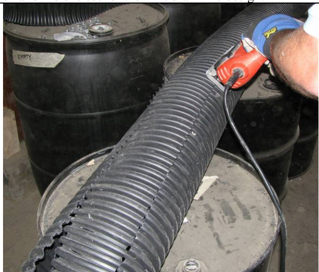
Figure 20. Cutting a 3-in. “walkway” in the 15 cm flex pipe with jigsaw (note: a jigsaw works best for this task).
