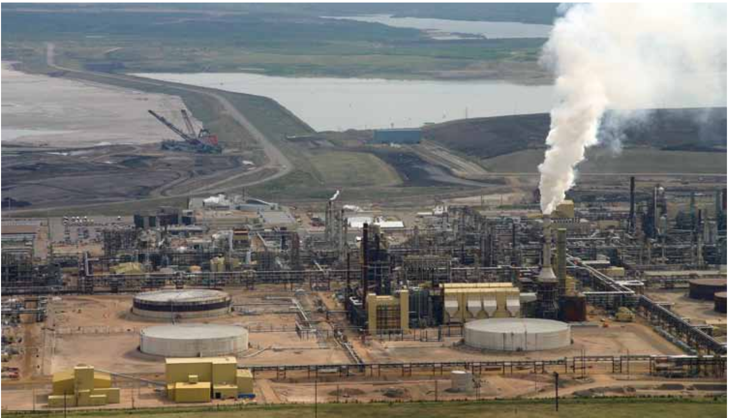
Top: The Athabasca River snakes south of Fort McMurray in Alberta, Canada. Above: Syncrude processing facility and upgrader mars the boreal landscape.
